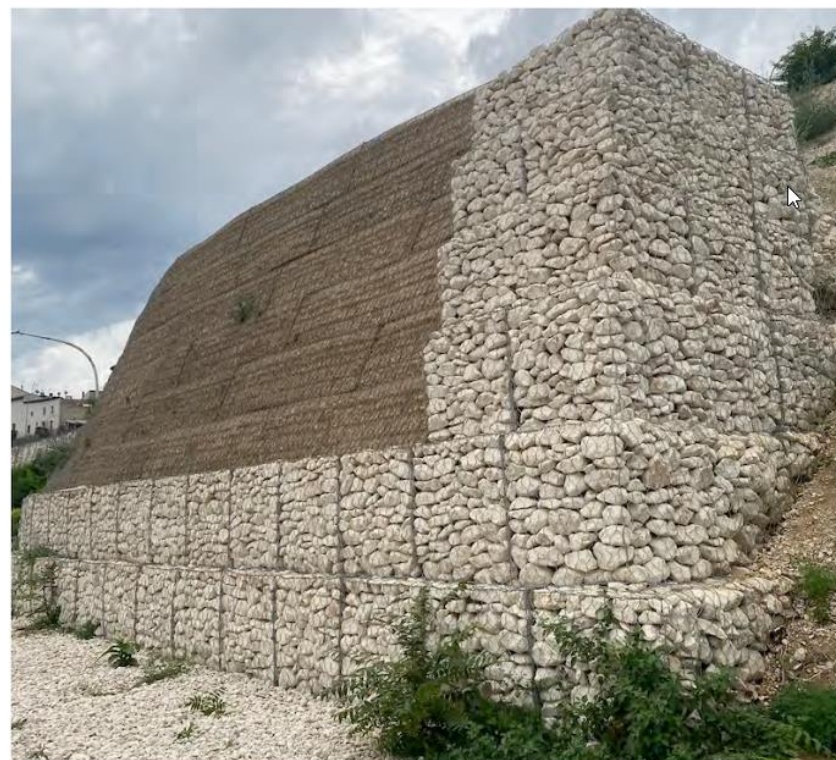
Gabion walls are used to control erosion. Photo courtesy of Michel Di Tommaso.
