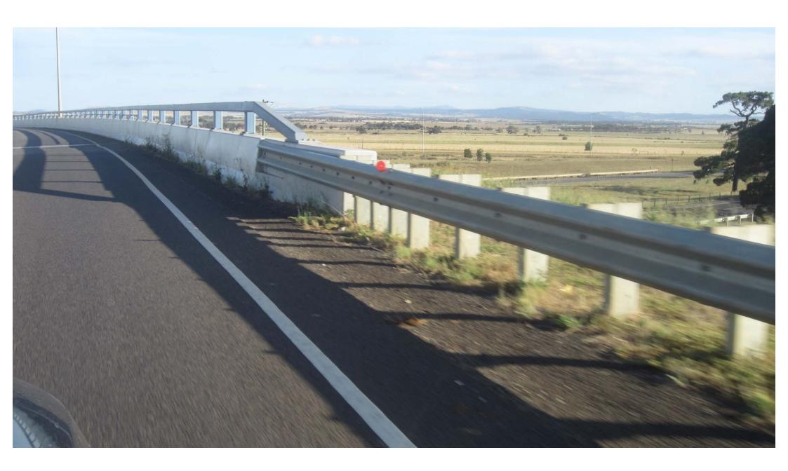
Unsafe! A safe terminal is needed to avoid spearing vehicles. Very unsafe!
