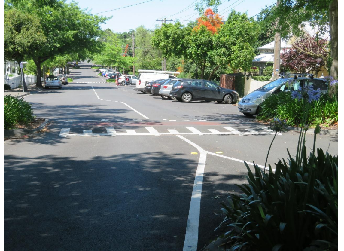
Vertical displacement
