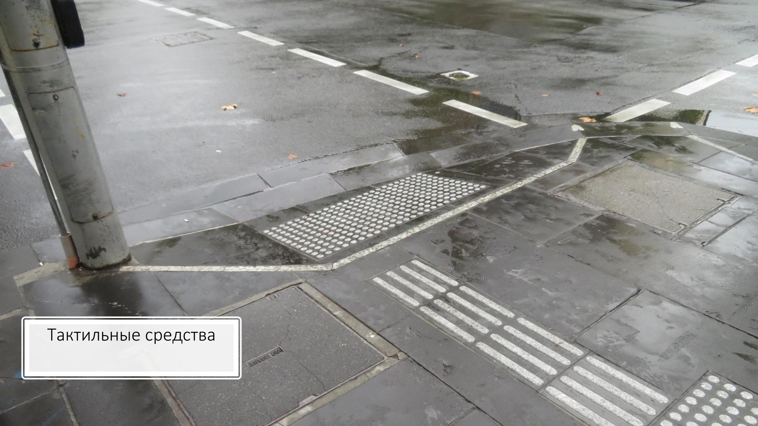
A photograph of a wet city street. In the foreground, there is a sidewalk made of large, dark grey tiles. On the sidewalk, there are two types of tactile paving: a rectangular mat with a grid of small white dots and a long, narrow strip with a series of raised white bars. To the left, a vertical metal pole stands on the sidewalk. The street itself is paved with asphalt and has several white dashed lines marking crosswalks. A manhole cover is visible in the lower-left corner of the sidewalk.
