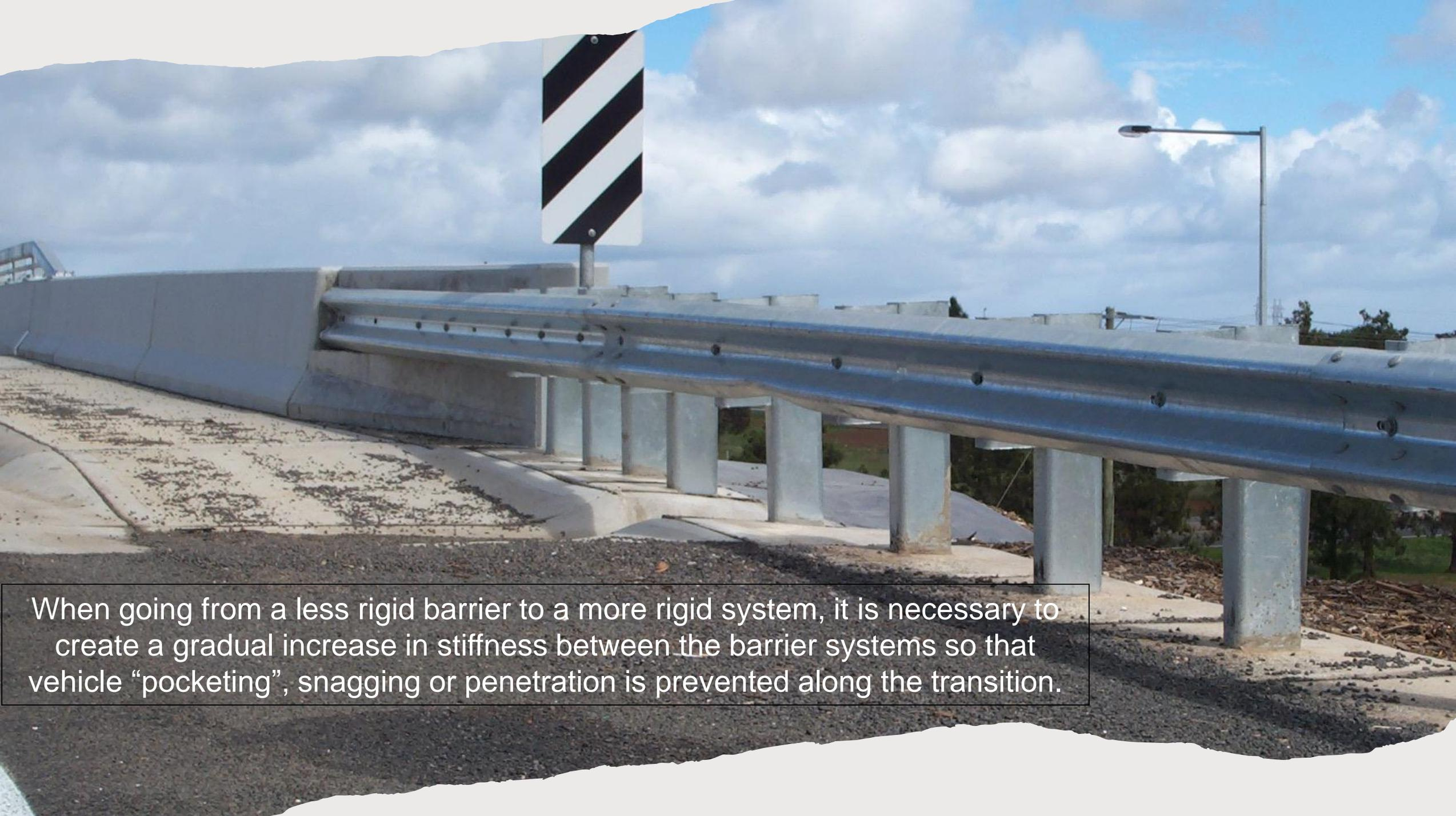
When going from a less rigid barrier to a more rigid system, it is necessary to create a gradual increase in stiffness between the barrier systems so that vehicle “pocketing”, snagging or penetration is prevented along the transition.
