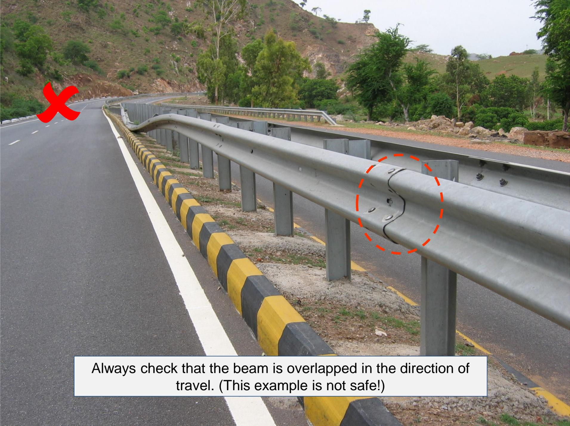
Always check that the beam is overlapped in the direction of travel. (This example is not safe!)
