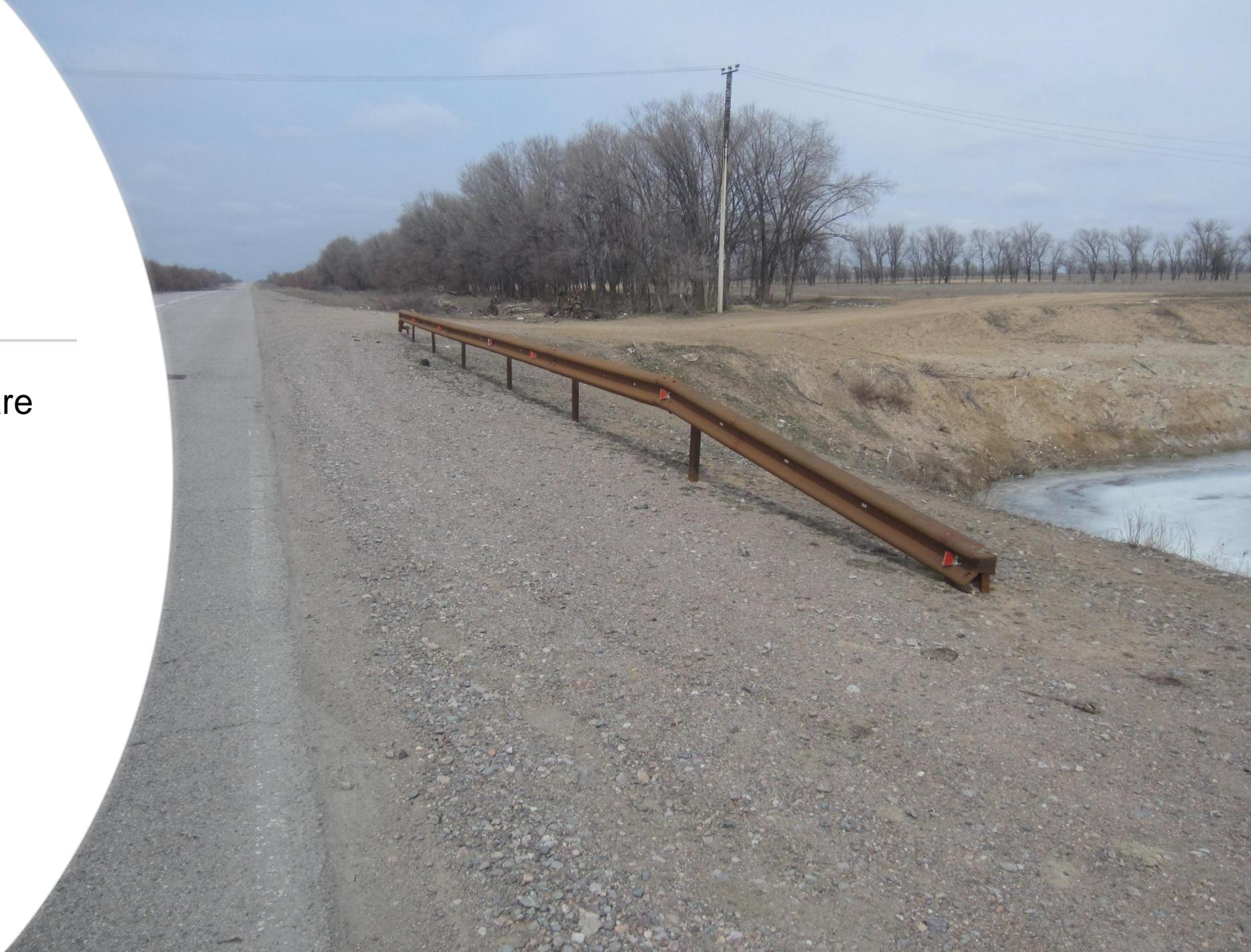
Sloped end treatments are dangerous. If struck, the vehicle may become airborne or overturn.
