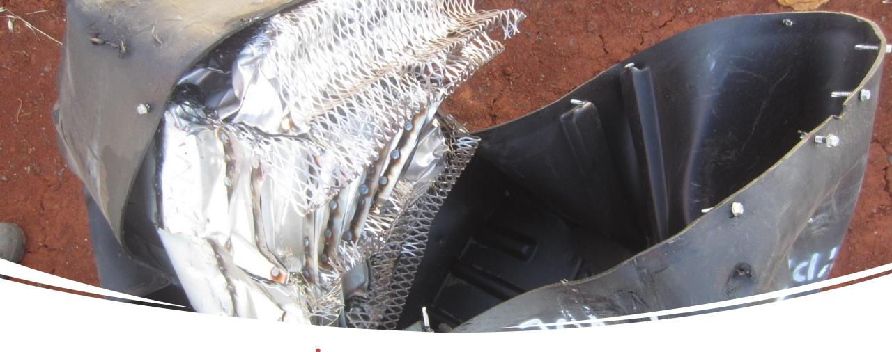
Inside an impact attenuator cartridge
