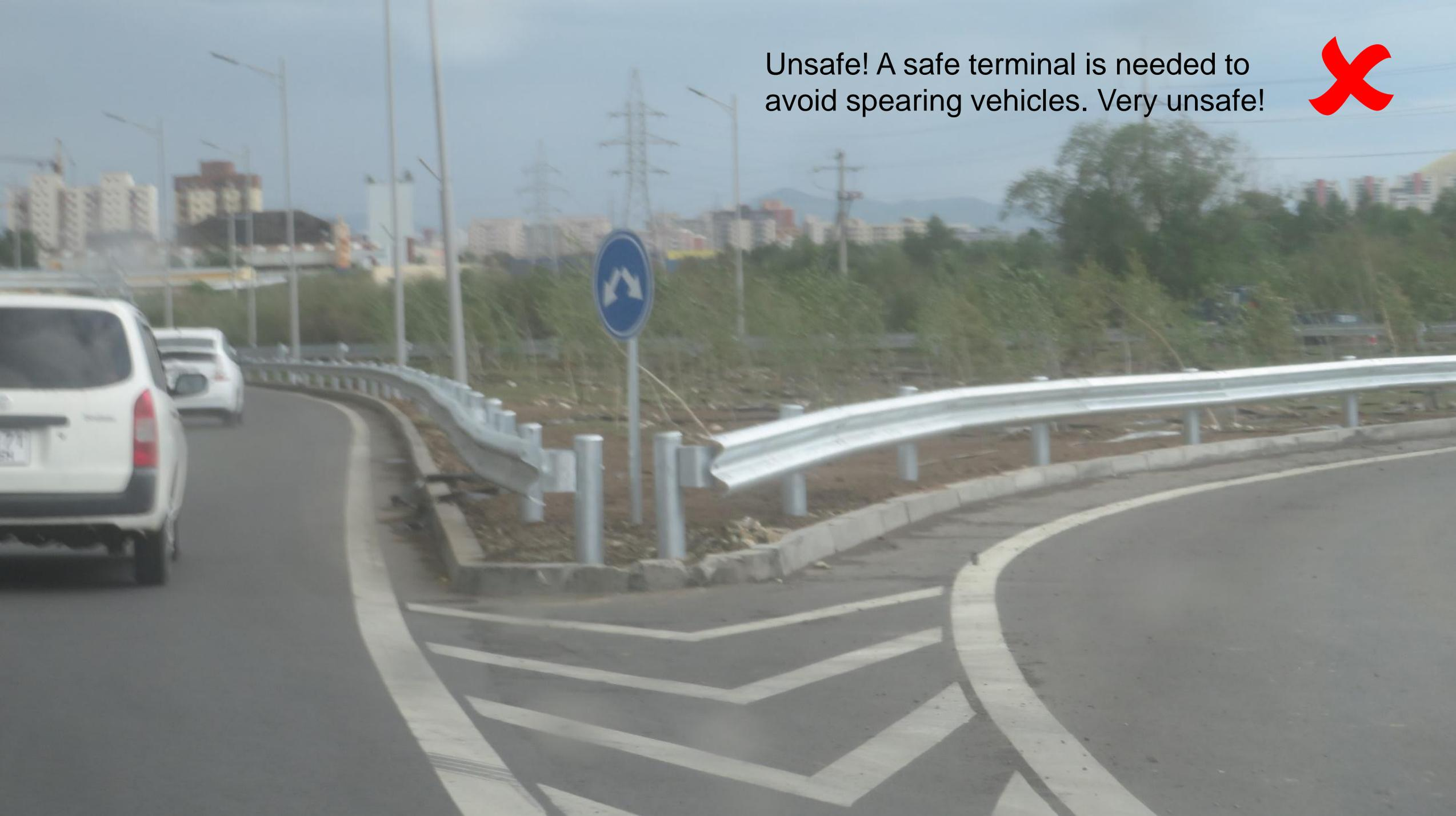
Sloped end treatments are dangerous. If struck, the vehicle may become airborne or overturn.
