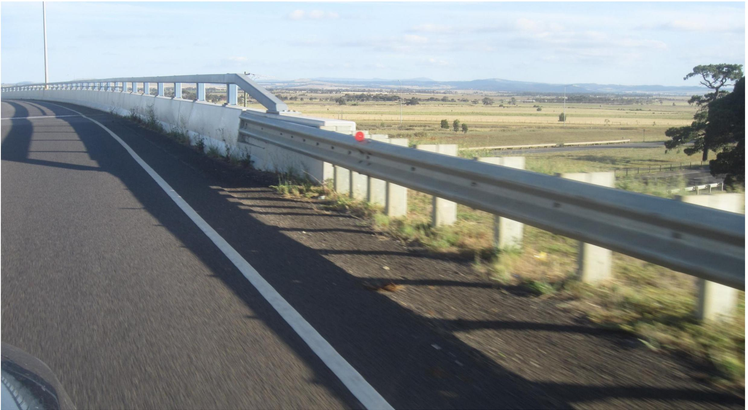
Unsafe! A safe terminal is needed to avoid spearing vehicles. Very unsafe!
