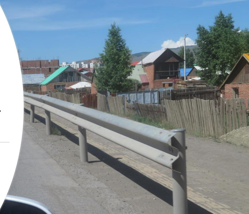
End treatments are necessary to avoid penetration into the vehicle
