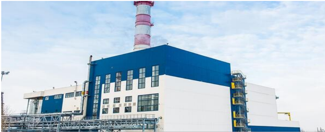
Kolpino CHP Plant – St. Petersburg, Russia
