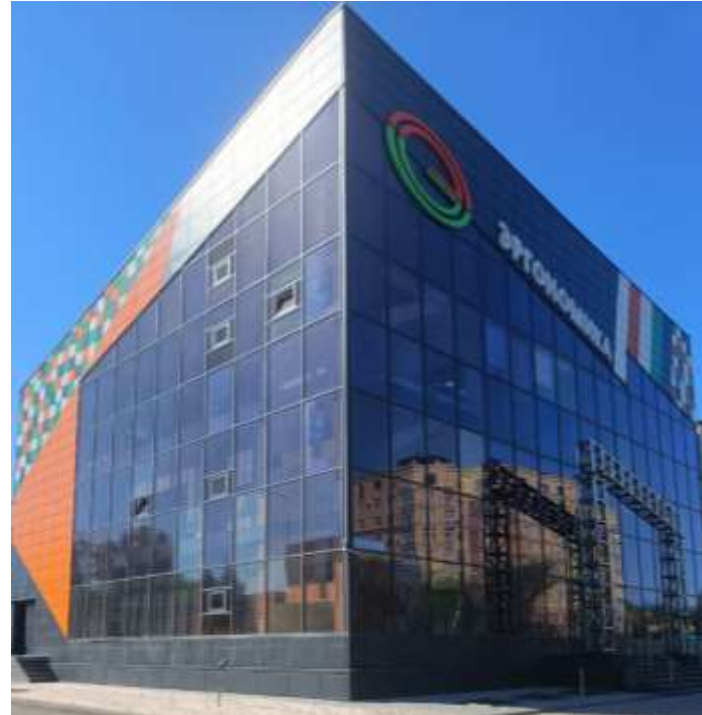
South facade - glazing
