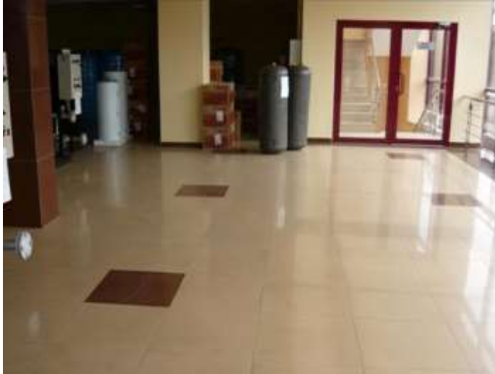
Underfloor heating - 85% of the load
